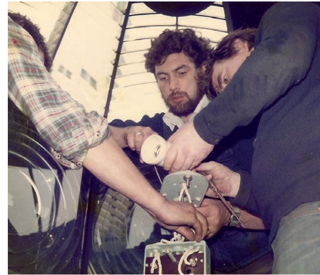
Electrification of the East Light from an incandescent burner, 1981, courtesy of Paddy Cleary
